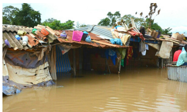
Flooding for inside Bayelsa Community
