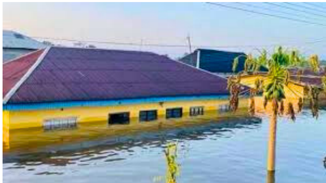
Flooding for Akinima, Rivers state
