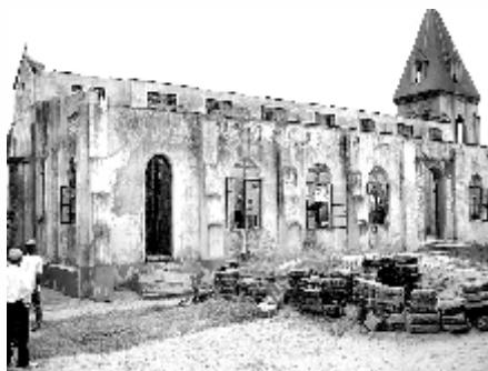
Destroyed Church building, Tombia
